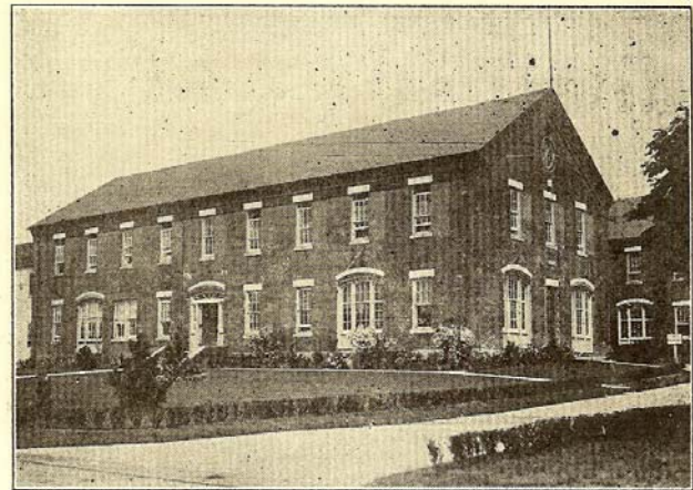
ADMINISTRATIVE BUILDING NO. 1.
